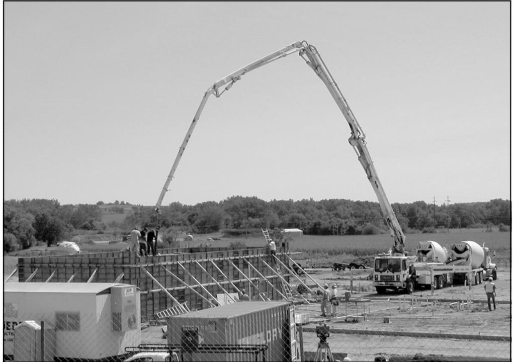
**Construction update:** On September 7th, construction crews poured the concrete walls for the new vault and head end portion of the HMU Operations Center.
