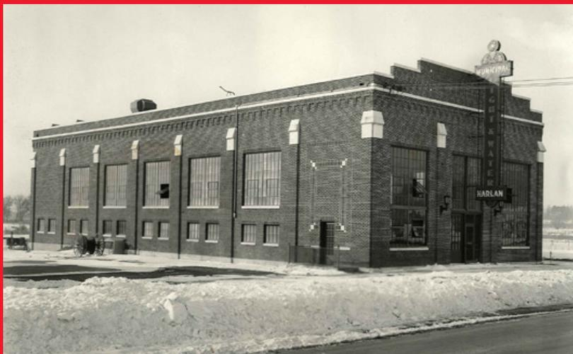
**As the demand for electricity grew, new diesel powered generators were added to the plant. An addition was added to the south end of the plant. Compare the length of the plant to the left to the original layout above. The light plant was used for storage after the generators were removed in the late 1980's.**
